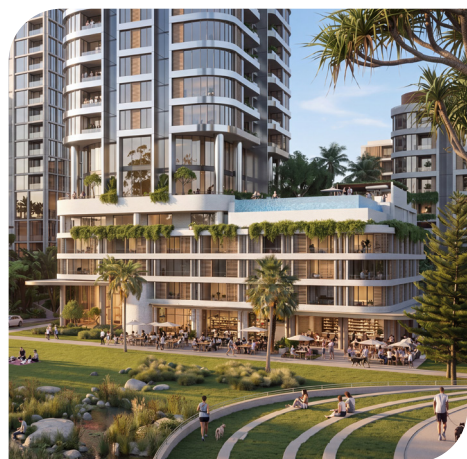
Montague Road (former Visy)
